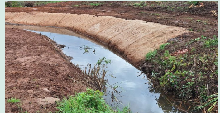
Existing watercourse where fish rescue was completed
