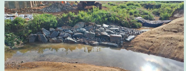
Upstream end of watercourse, old section was maintained as an ecological feature, re-graded to backfall. A riprap bund was installed to guide the main flow of water, with a 300mm diameter pipe was installed to allow passage of fish to the between the old and new sections of watercourse.
